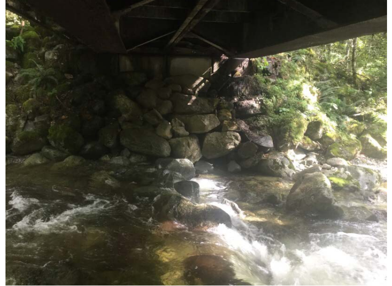
Left Bank Abutment when facing downstream
