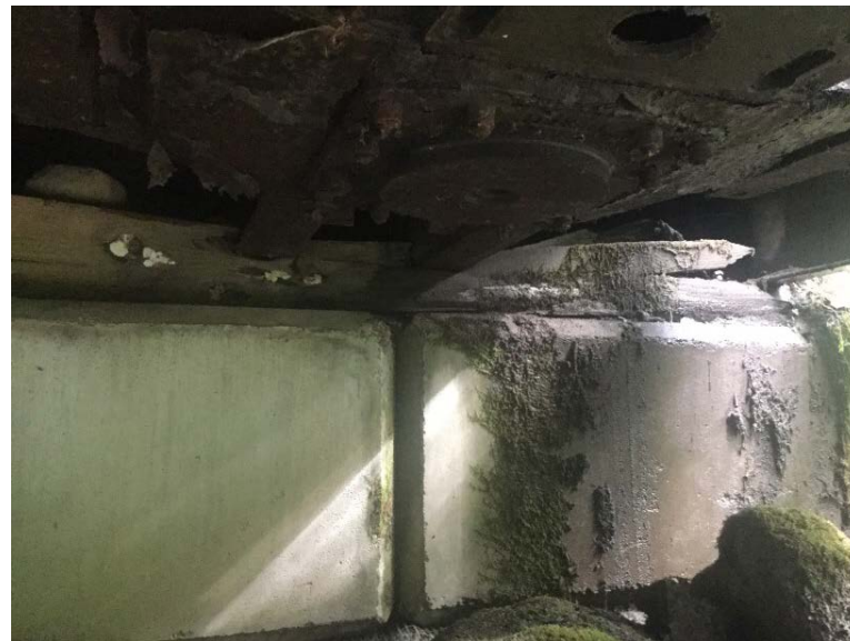
Left bank sill
