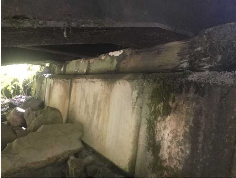
Right Bank Abutment when facing downstream
