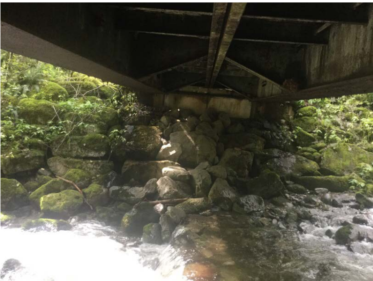
Right Bank Abutment when facing downstream
