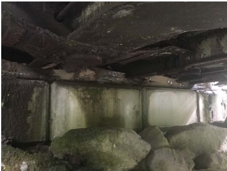
Left bank sill
